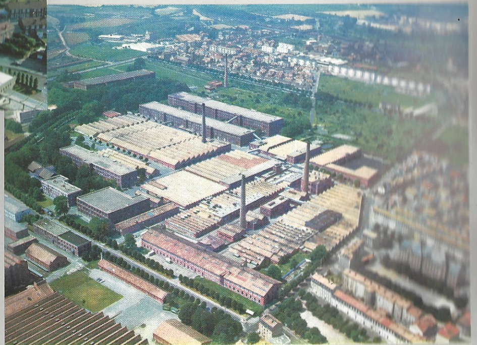
MULHOUSE'S FACTORY - Aerial view
